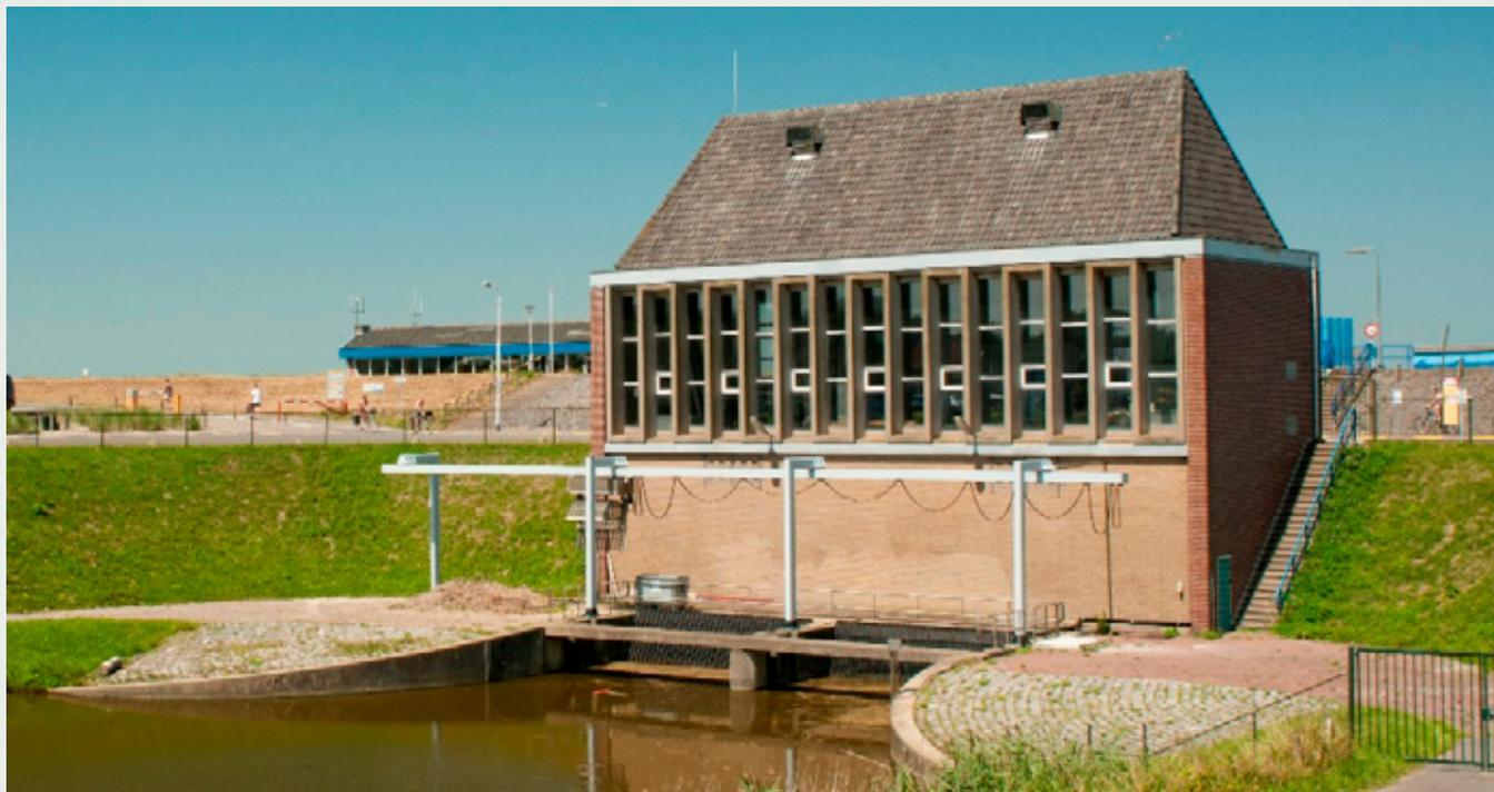
The polder pumping stations are responsible for 40% of the Scheldestromen Water Authority's energy consumption. De Dommel Water Authority has developed a new control system, which is able to handle not only high and low water levels but also weather conditions. This results in energy savings and more efficient drainage, which reduces the likelihood of flooding. It is also beneficial to fish migration, while it will counter soil salinisation and dehydration as well.
